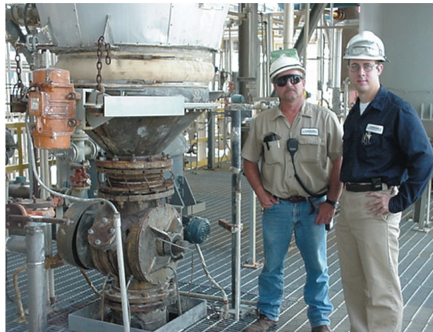
Charlie Covington, Albemarle's complex maintenance coordinator (left), and Jason Bitting, senior mechanical excellence engineer, check the seal for leakage and find none.
